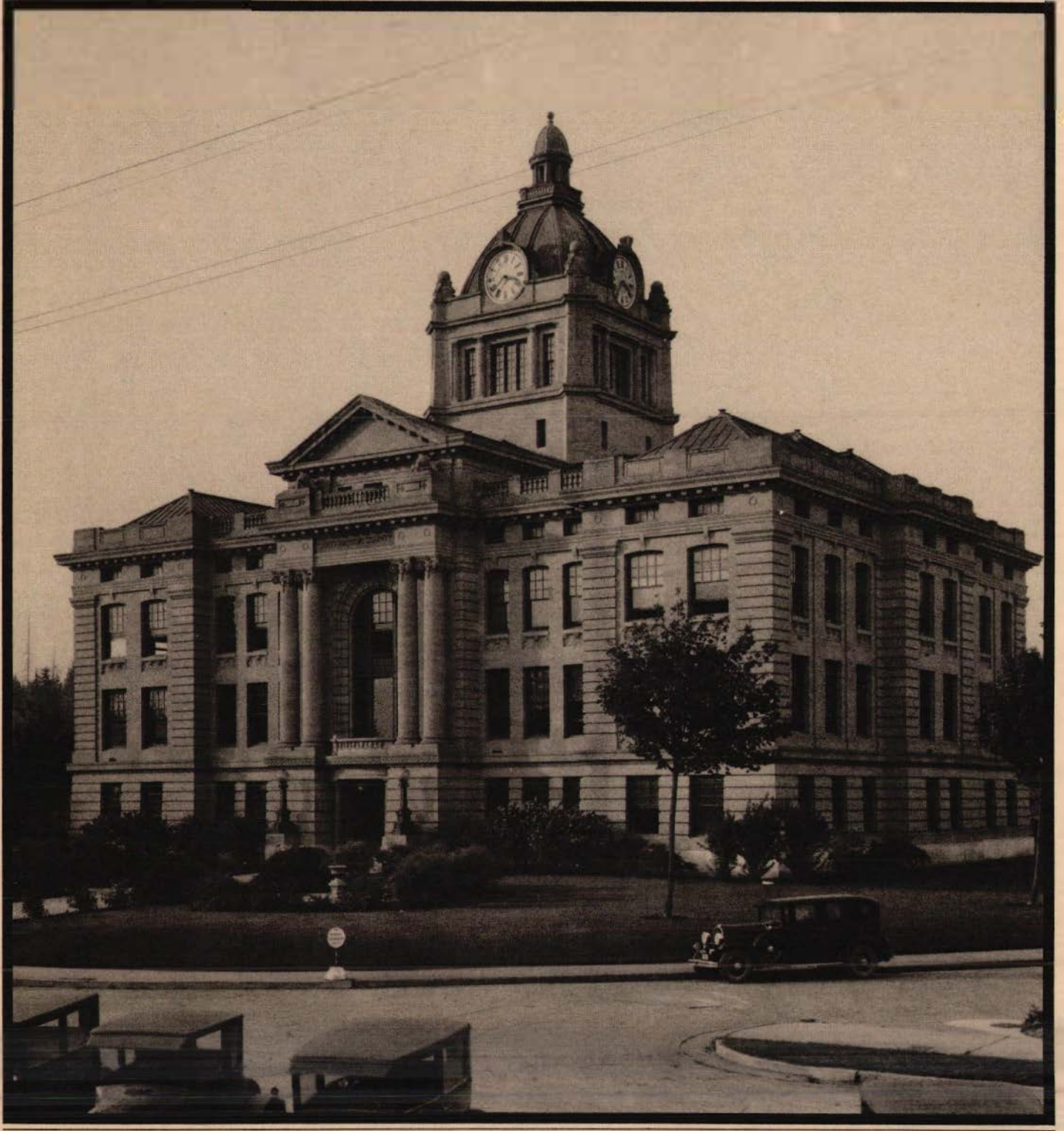
Grays Harbor County Courthouse
