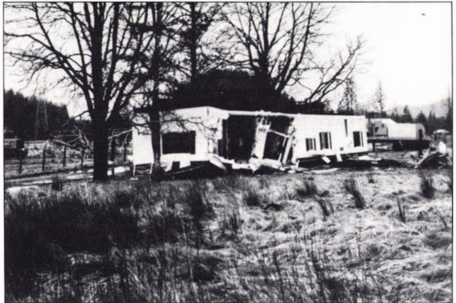
An overturned mobile home near Enumclaw destroyed during the windstorm of December 24, 1983.
