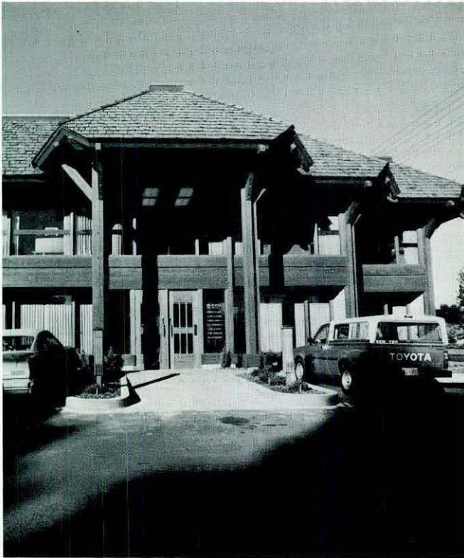
Main entrance of Lyon Law Office is adjacent to ample parking. Extension of second floor in rear provides covered parking for staff.
