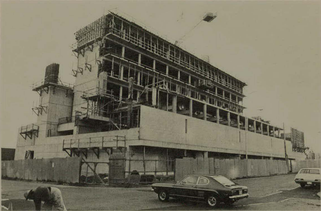
N.E. corner; library reading room in lower foreground.
